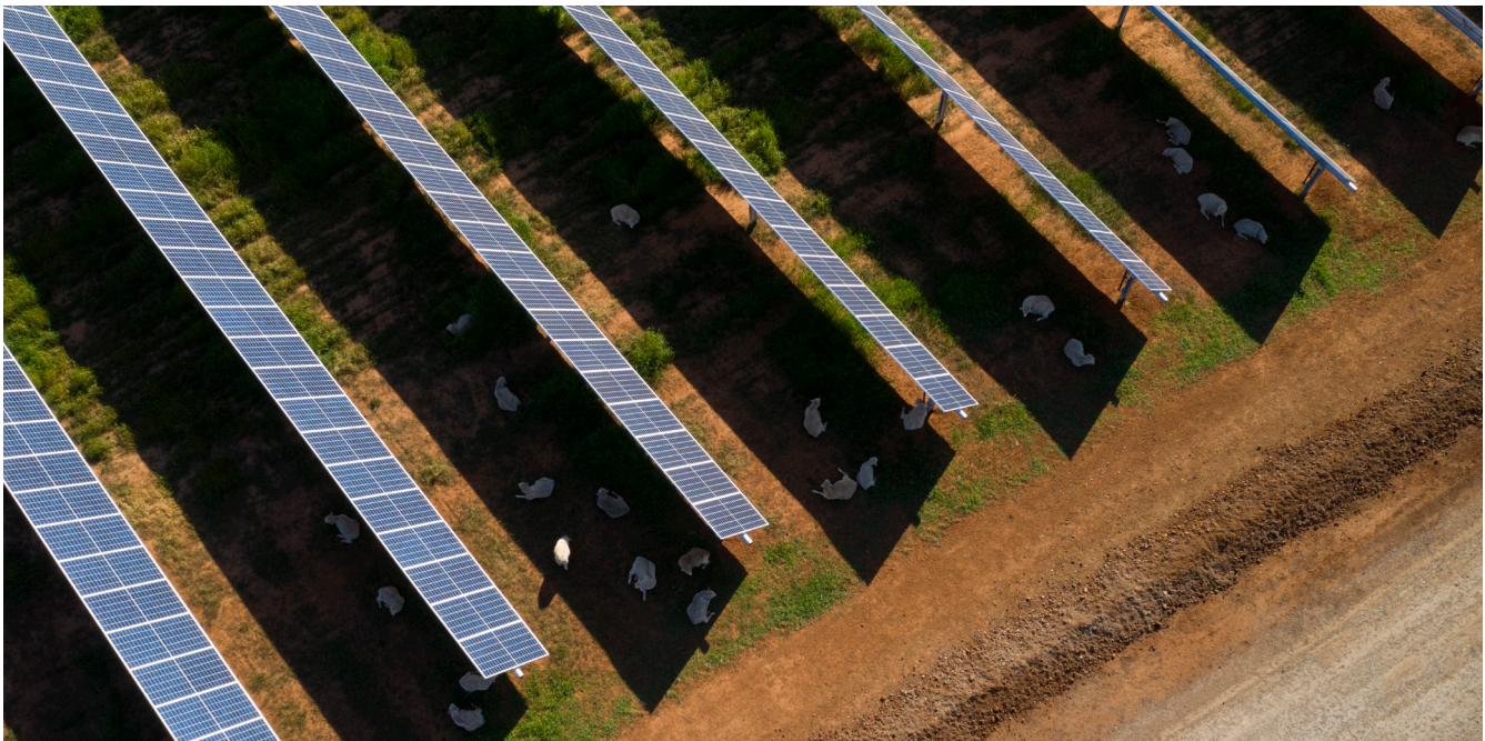
Finley Solar Farm, NSW
