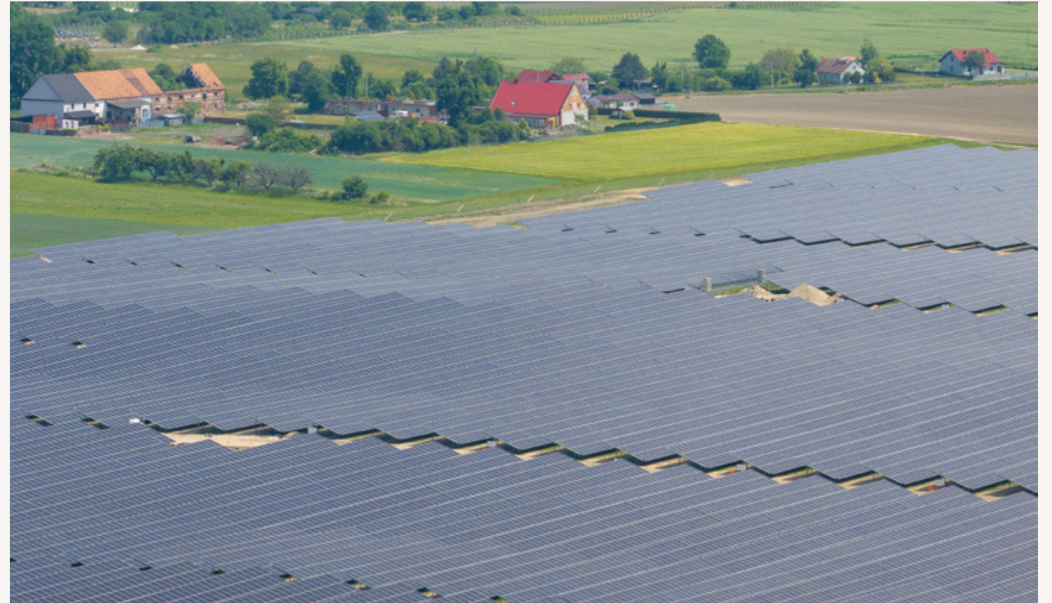
Rutki: a 100 MW solar farm located in Niemodlin municipality in the Opolskie region.
