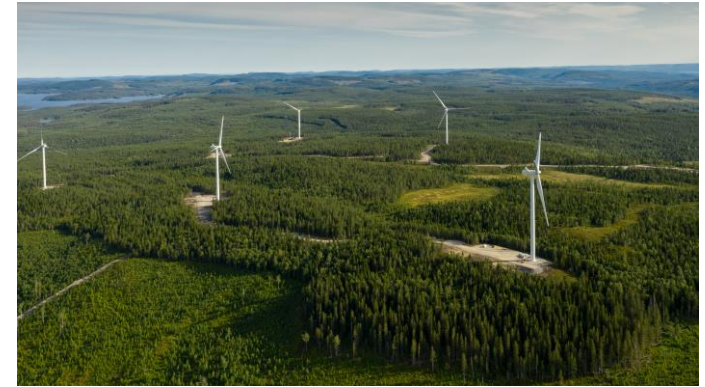
Wind farm handed over
